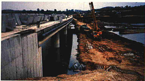
The construction of the Express Rail Link was interfaced with the wetland development.
