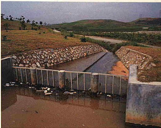
Gross pollutant traps have to be cleaned regularly so that they can capture debris and other litter effectively
