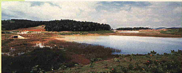
The two cells of Upper Bisa occupy a total of 236 hectares. They are south of the lake and discharge water directly into Putrajaya Lake
