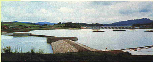
The Central Wetlands is one large 509 hectare cell, where water from the four wetlands (Upper Bisa excluded) is collected before being discharged into the lake
