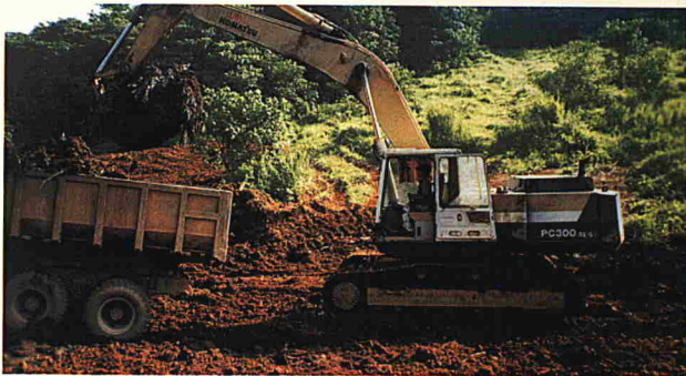
Earthworks was aimed at achieving a balance of cut and fill
