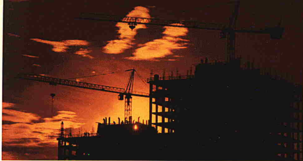
Construction activity resulted in increased run-off that had to be mitigated
