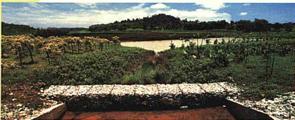
Upper East Wetlands, with three cells, is relatively small with an area of 158 hectares (Cell UE3 above)
