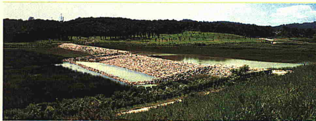
A cell in the Upper Wetlands, with an extensive macrophytic zone. Note the ZII encircling the submerged area, which is divided by a weir that regulates water flow.
