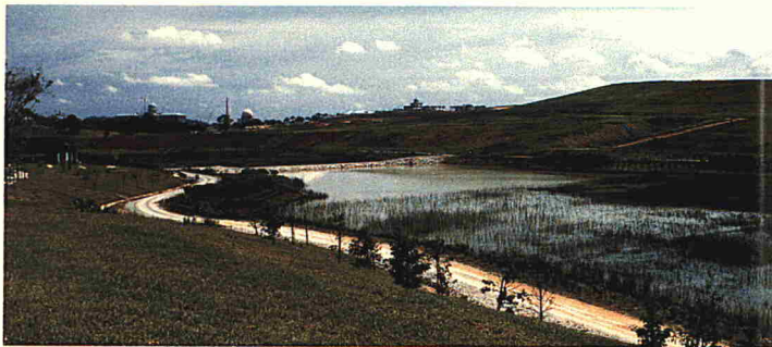
Wetland cells can be accessed by a network of maintenance tracks
